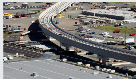
Dulles Guideway Track
